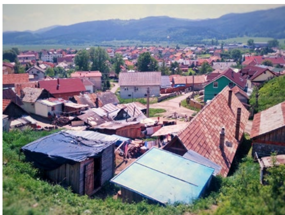
Hrabušice – on the outskirts of the village, a neighbourhood with partly informally built homes in poor condition is inhabited mostly by Roma, while other Roma families live in more integrated parts of the village where housing conditions are better (©Sheena Keller)
